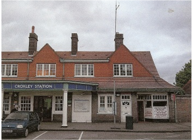
Frame No: 01 Location: Croxley Station Flat
